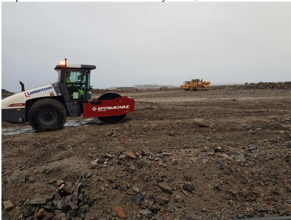
Figure 3. Tuesday morning, February 8, 2022. The testing has just begun.
