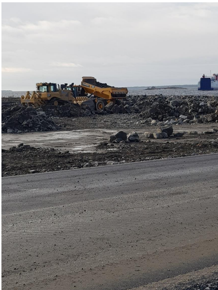
Figure 9. Filling of material in the exploitation area.
