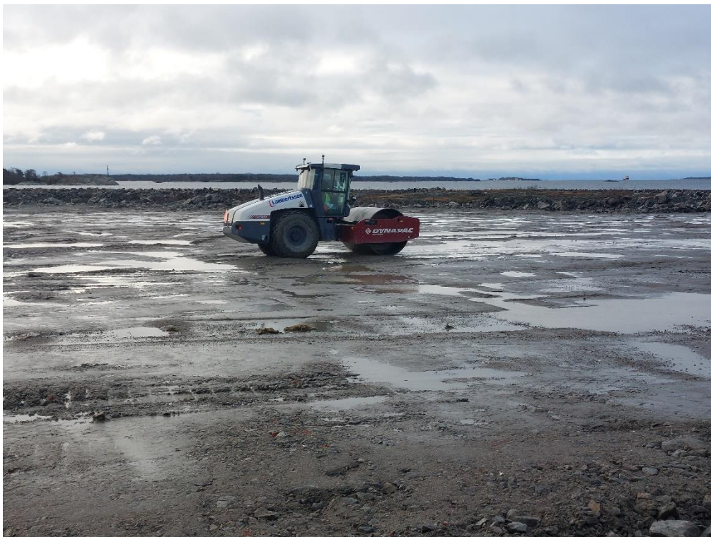
Figure 21. Day three week two, Eco Mode + Seismic on a quite wet surface.
