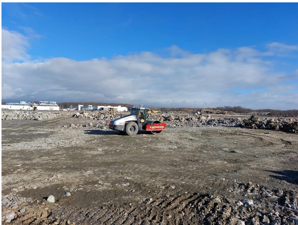
Figure 16. A view of the working roller.
