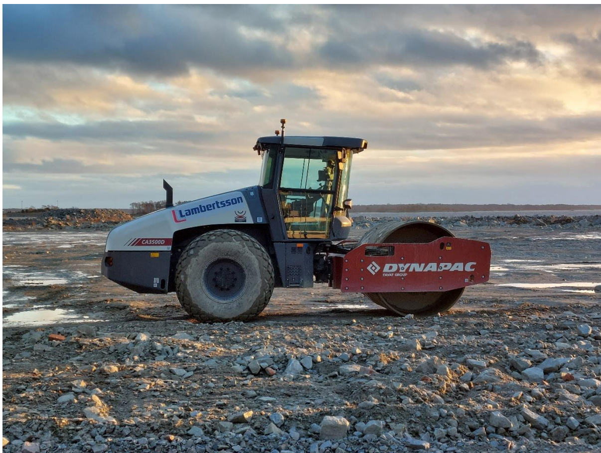
Figure 24. After work. The parked roller after the two weeks of testing at Verkö in Karlskrona, February 17, 2022.
