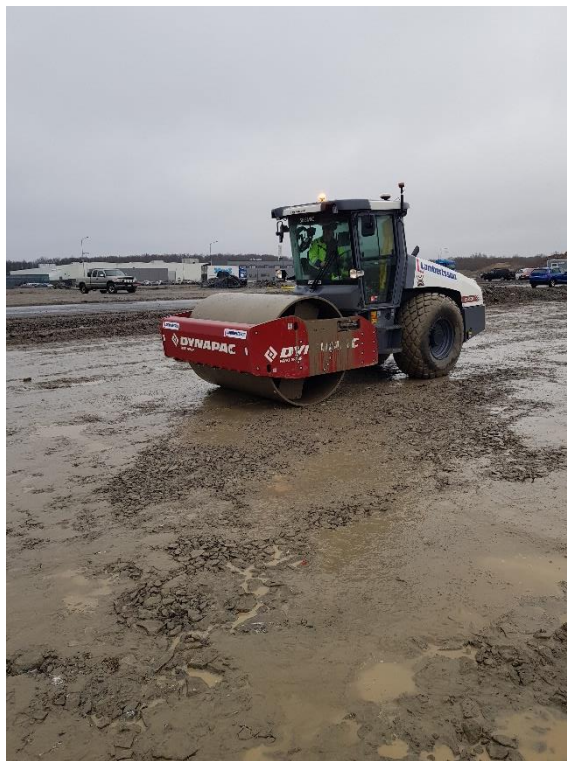
Figure 5. To the left: loose material. To the right: The roller on wet material with high fine content.
