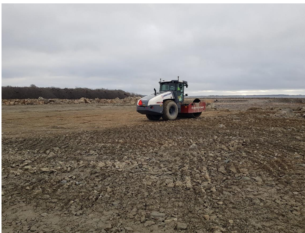
Figure 8. The roller in work day 2 with Eco mode.
