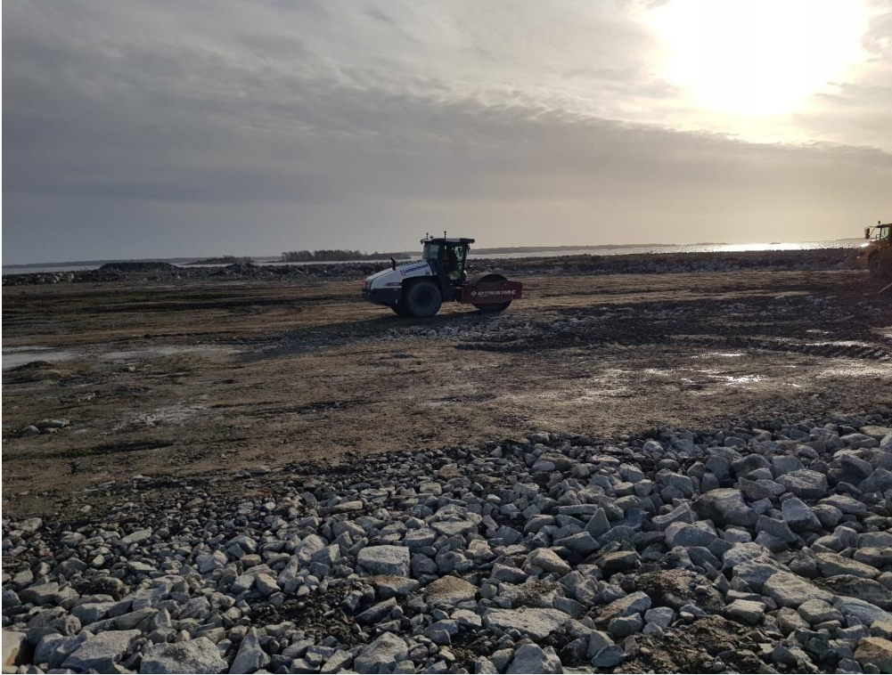
Figure 12. The roller in work during day 3, Eco mode + Seismic.
